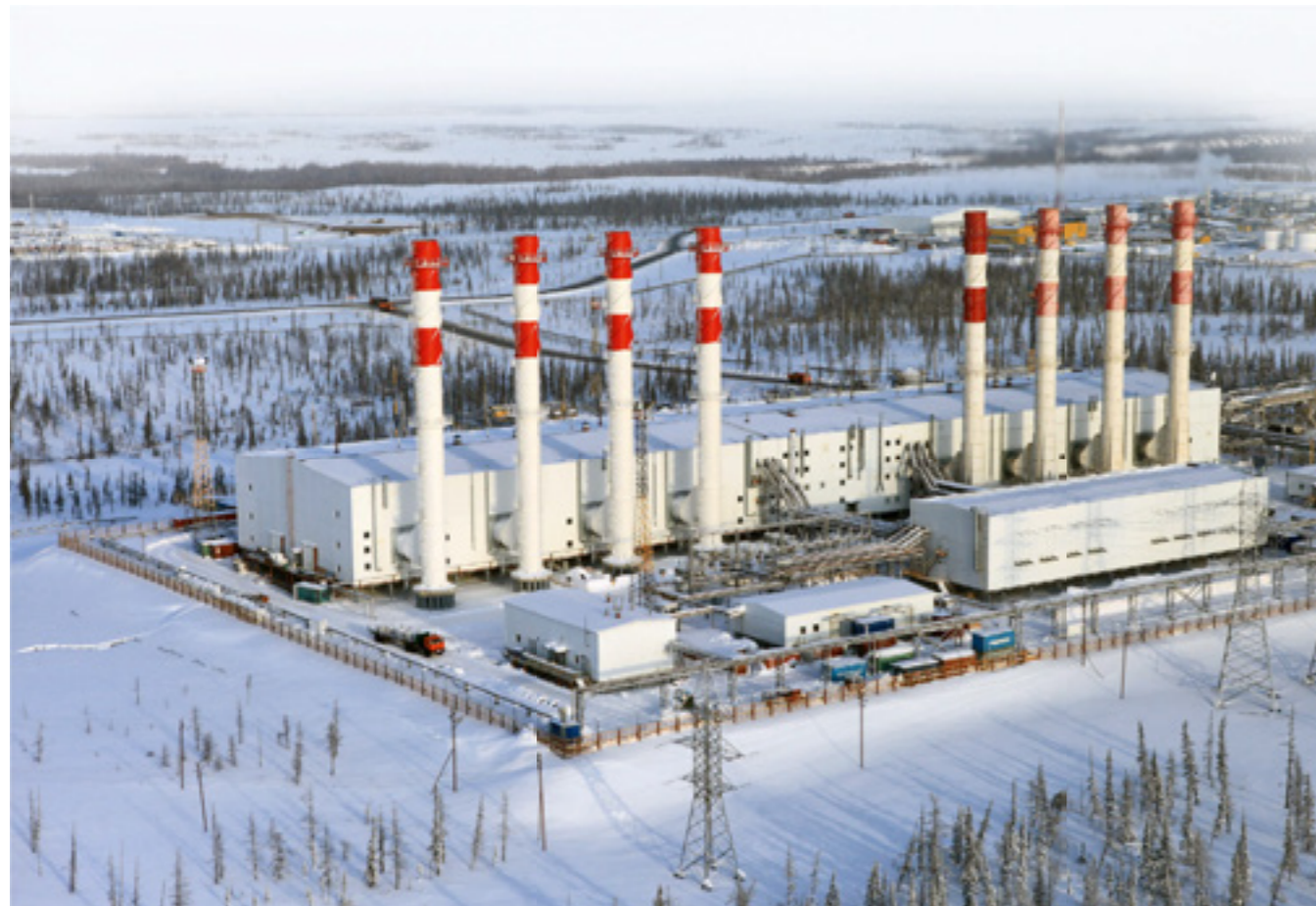
▲ Gas turbine power plant at the Vankor field
