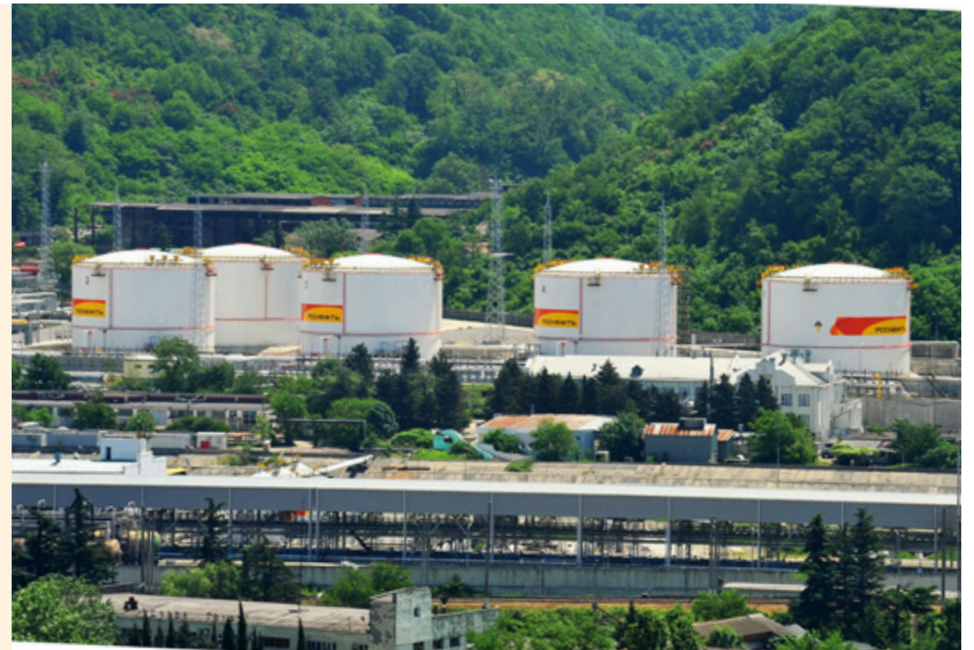
▲ The Tuapse Refinery
