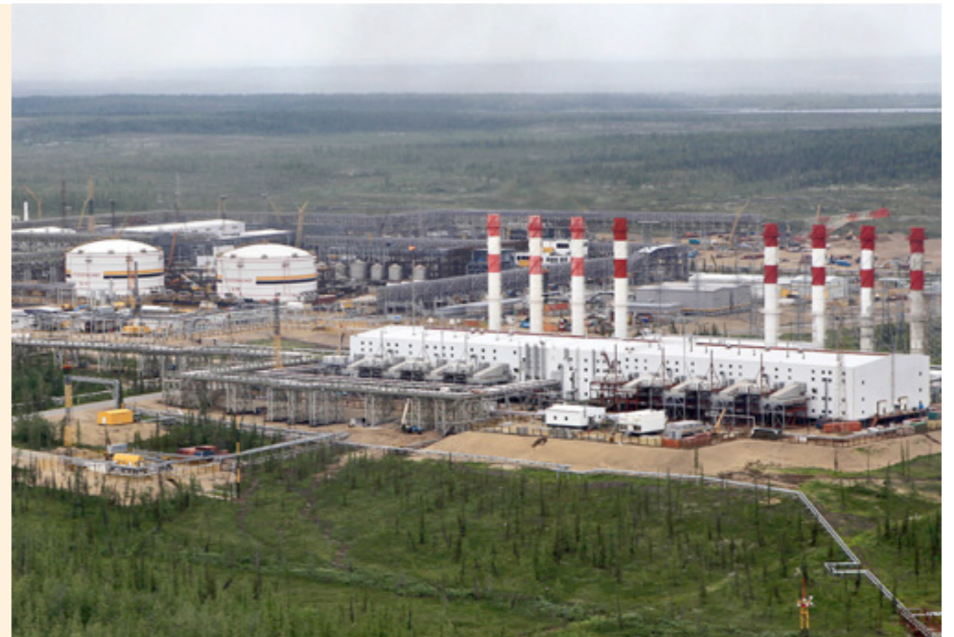
▲ Gas turbine power plant at the Vankor field
